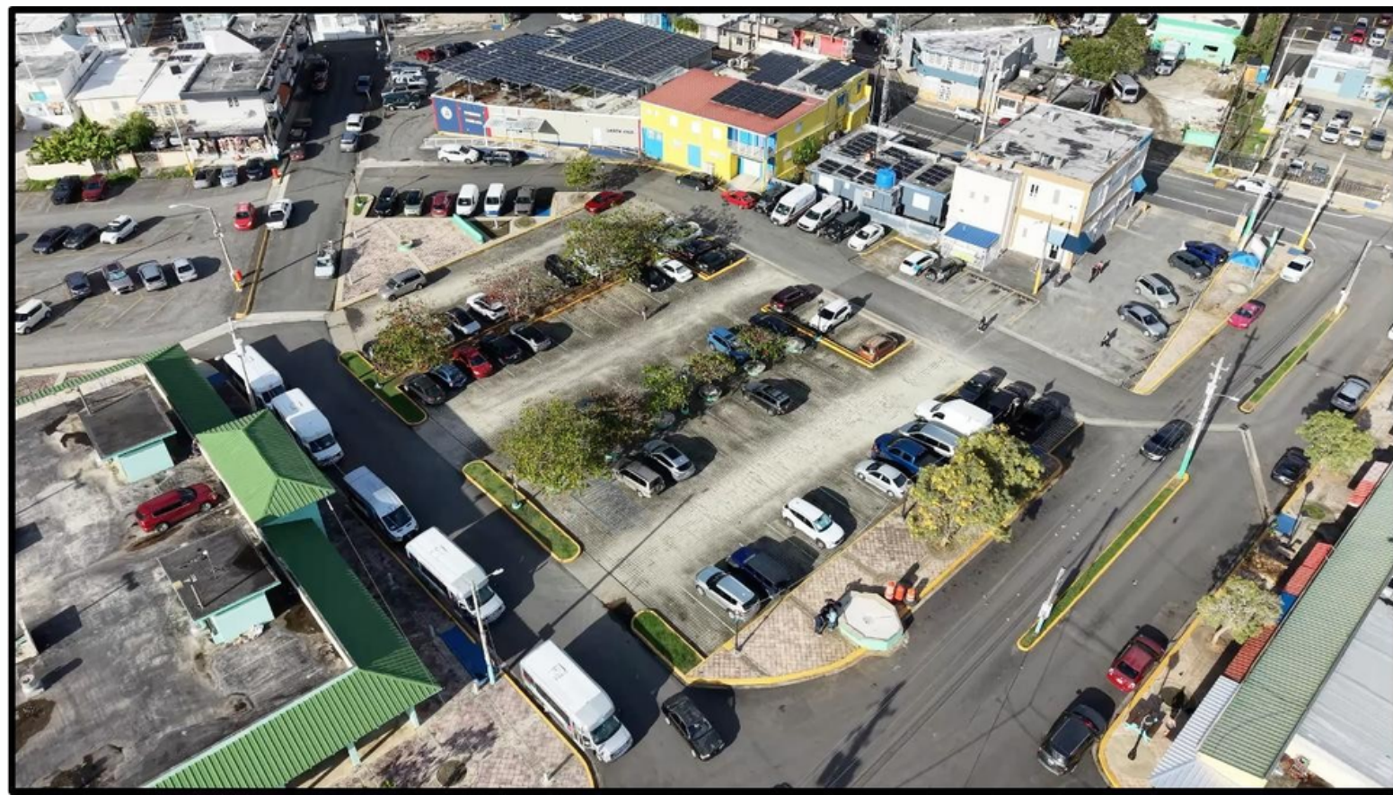
Figure 3: Existing Conditions Parking Lot
