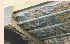
Figure 7 Partial Depth Repair
