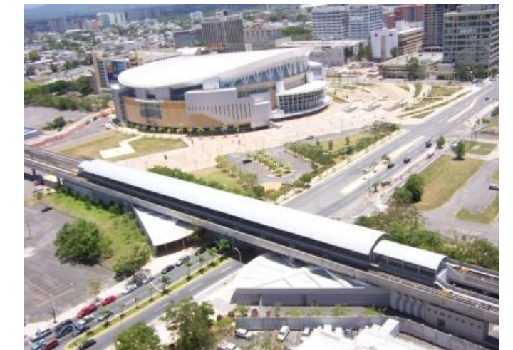
FIGURE 5: AERIAL PICTURE OF HATO REY STATION
