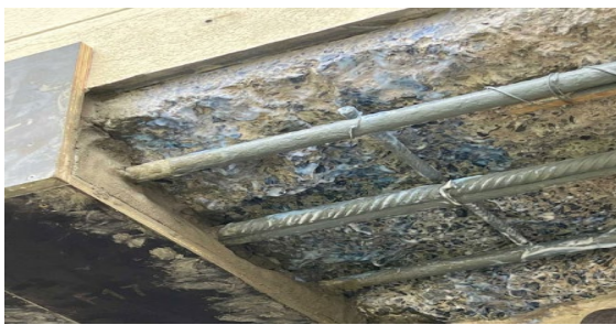
Figure 7 Partial Depth Repair
