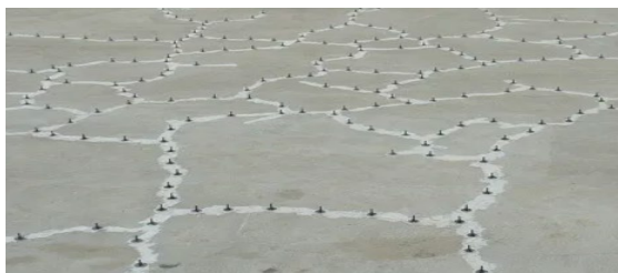
Figure 5 Crack Repair with Concrete Injection Grouting
