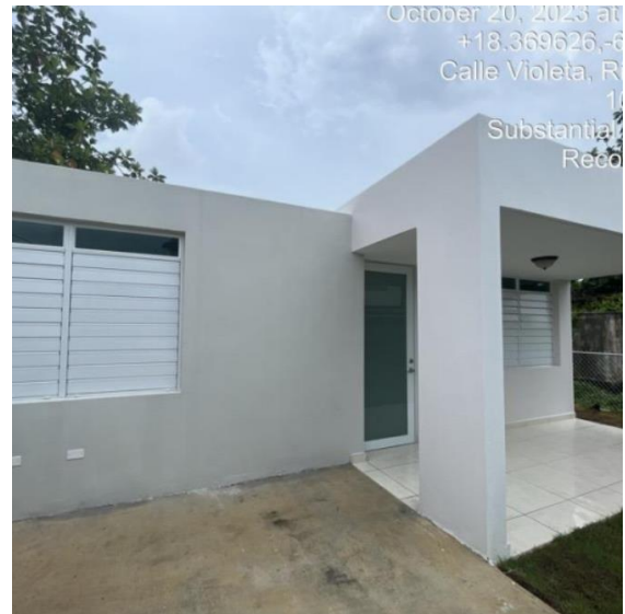
Figure 5 One-story 2-bedroom model home unit constructed at the original assessed site
