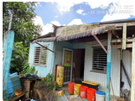
Figure 1 View of front elevation of the assessed property
