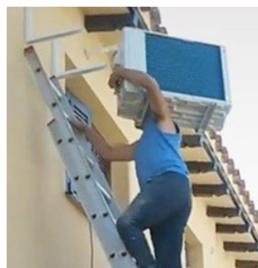
Figure 21 Carrying Condenser on shoulders.
