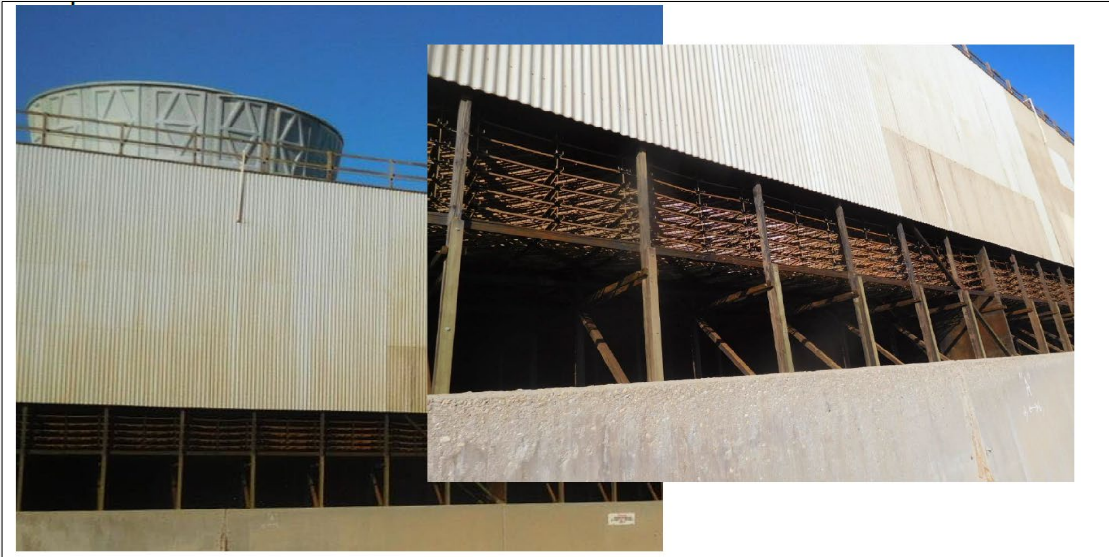
Figure 2 D- Bar splash fill installed in the air inlet section of the cooling tower cell after project implementation
