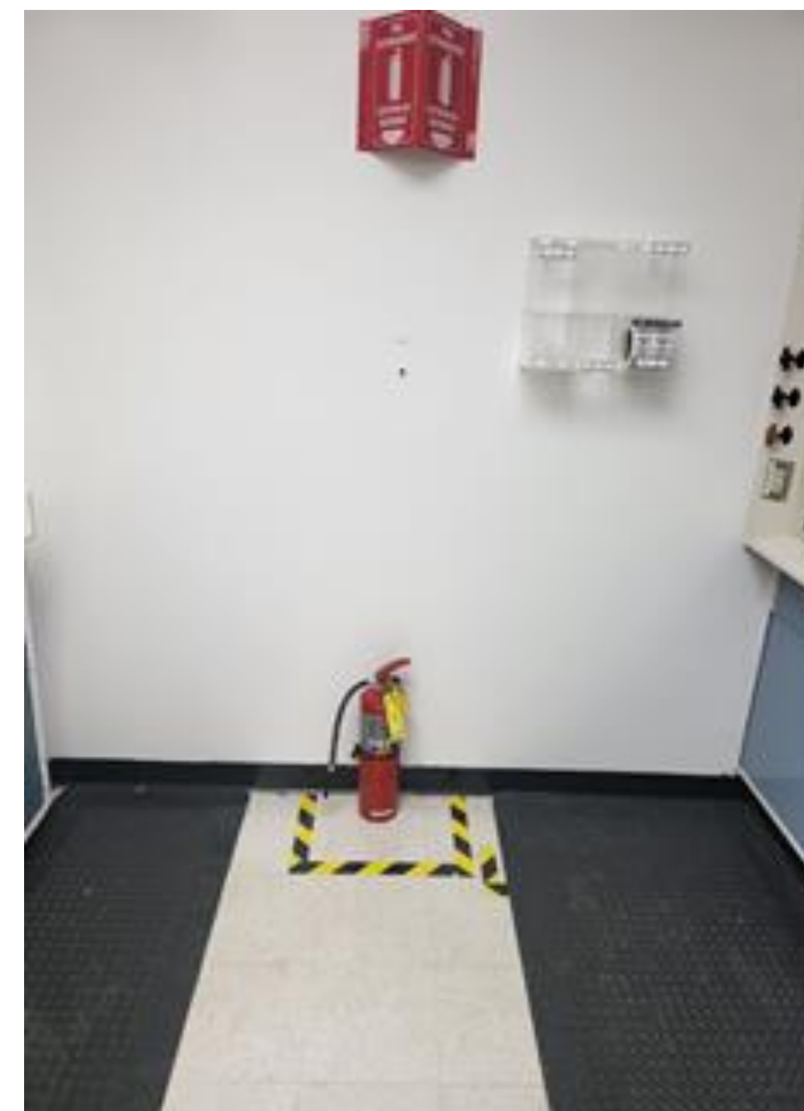
Figure 2 Non-Compliant Installation
