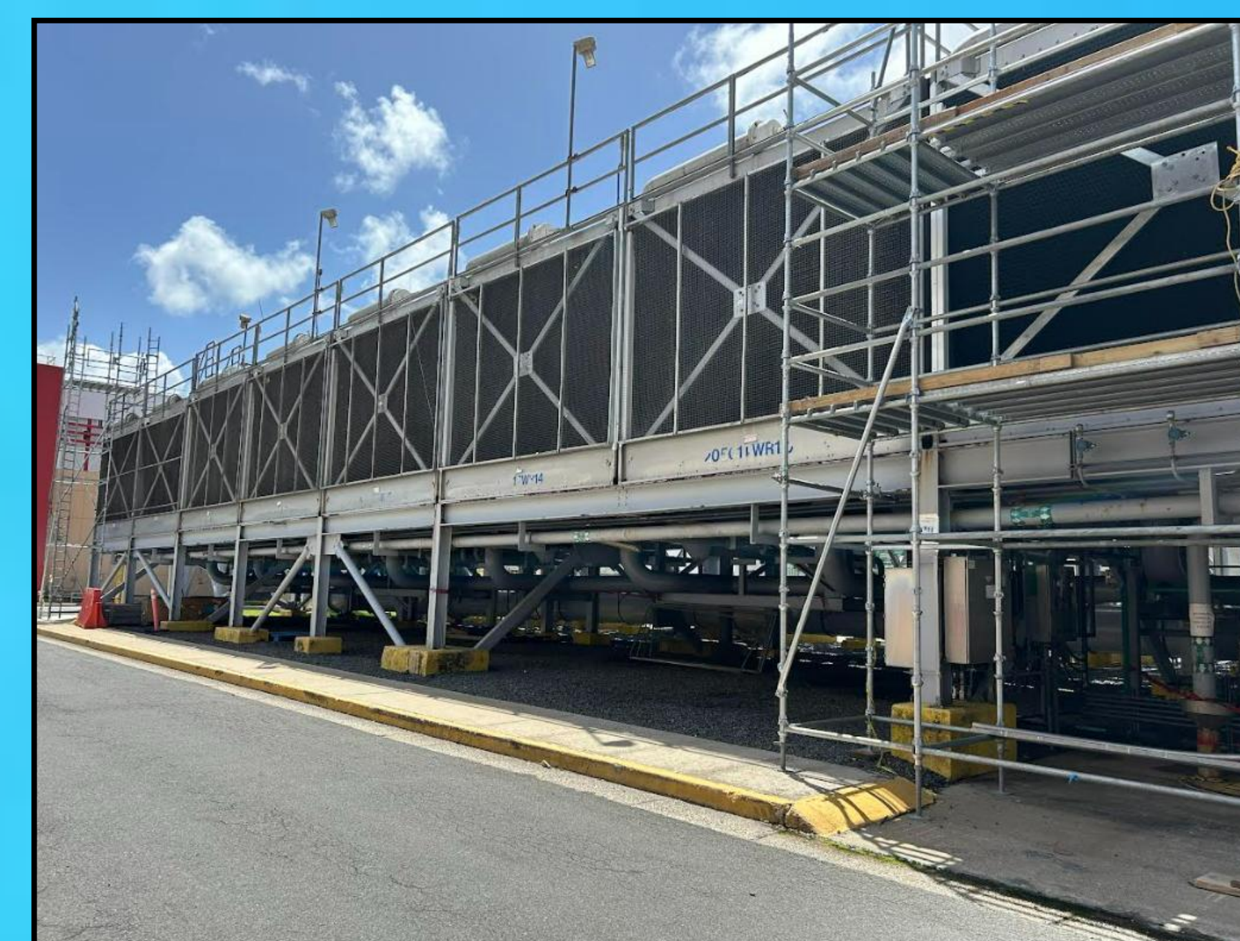
Figure 3: Central utility plant cooling towers with scaffolding installed for refurbishment.
