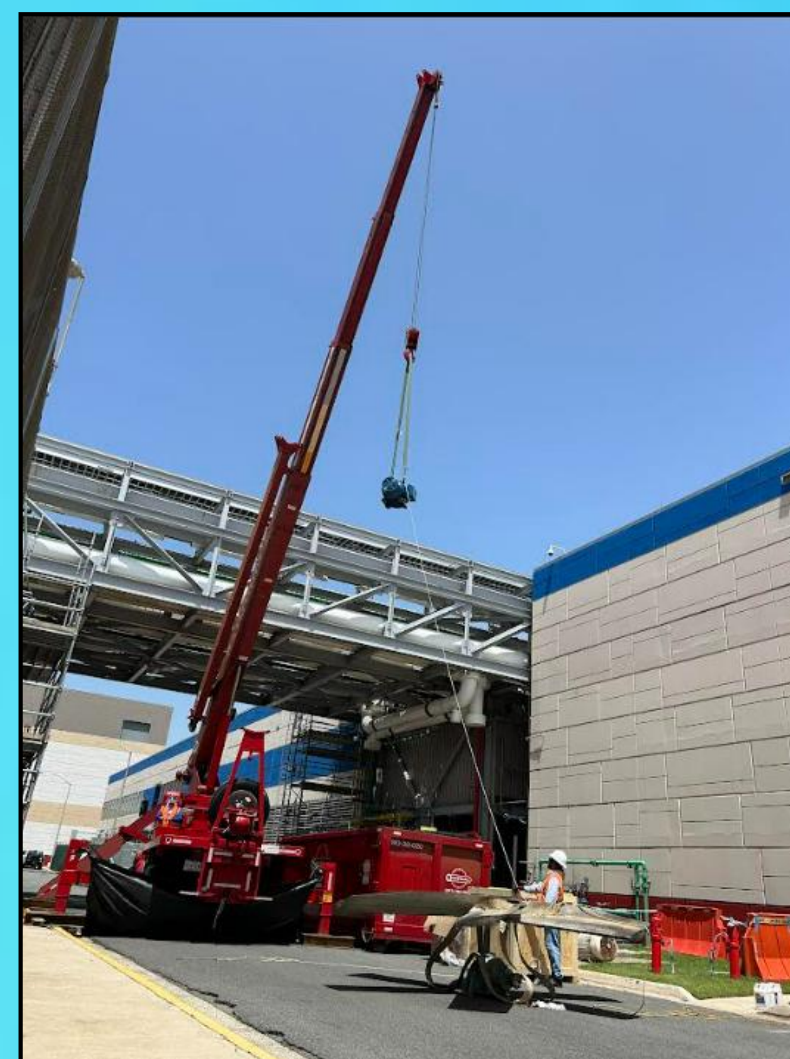
Figure 2: New motor installation with new transmission pending installation
