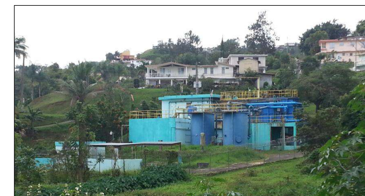
Fig. 2: Barrancas Filtration Plant
