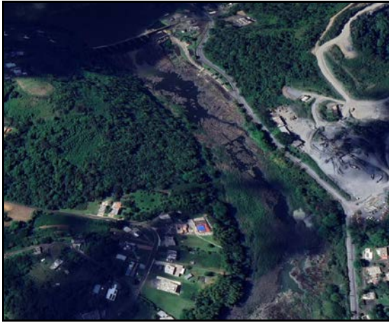
Figure 2 Exposed Riverbed Downstream Carraízo Dam
