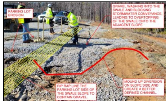
Figure 3 Erosion Control Inspection
