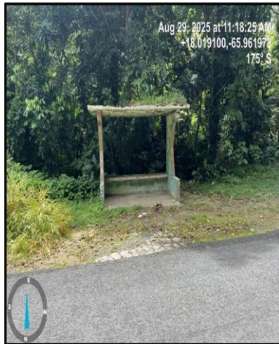
Figure 29 Current conditions at the bus stop. Note: Picture by Jean Calderón (2025).
