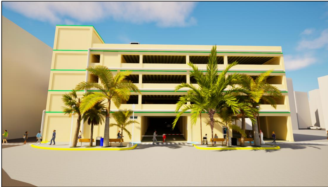
Figure 15. Front façade view of the multi-story parking structure.
