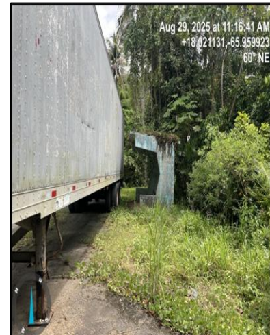
Figure 31 Current conditions at the bus stop. Note: Picture by Jean Calderón (2025).
