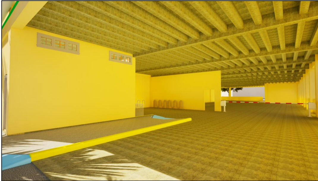
Figure 19. Bus entrance view of the multi-story parking structure.
