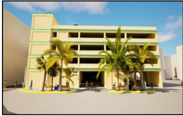
Phase 1- Multi-Story Parking Structure
