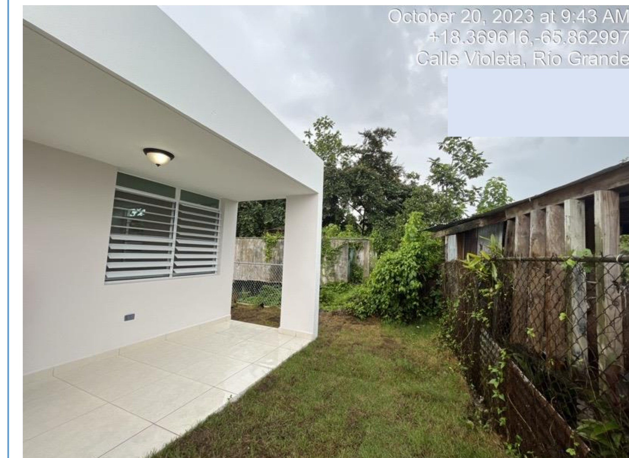
Figure 5. One-story 2-bedroom model home unit constructed at the original assessed site
