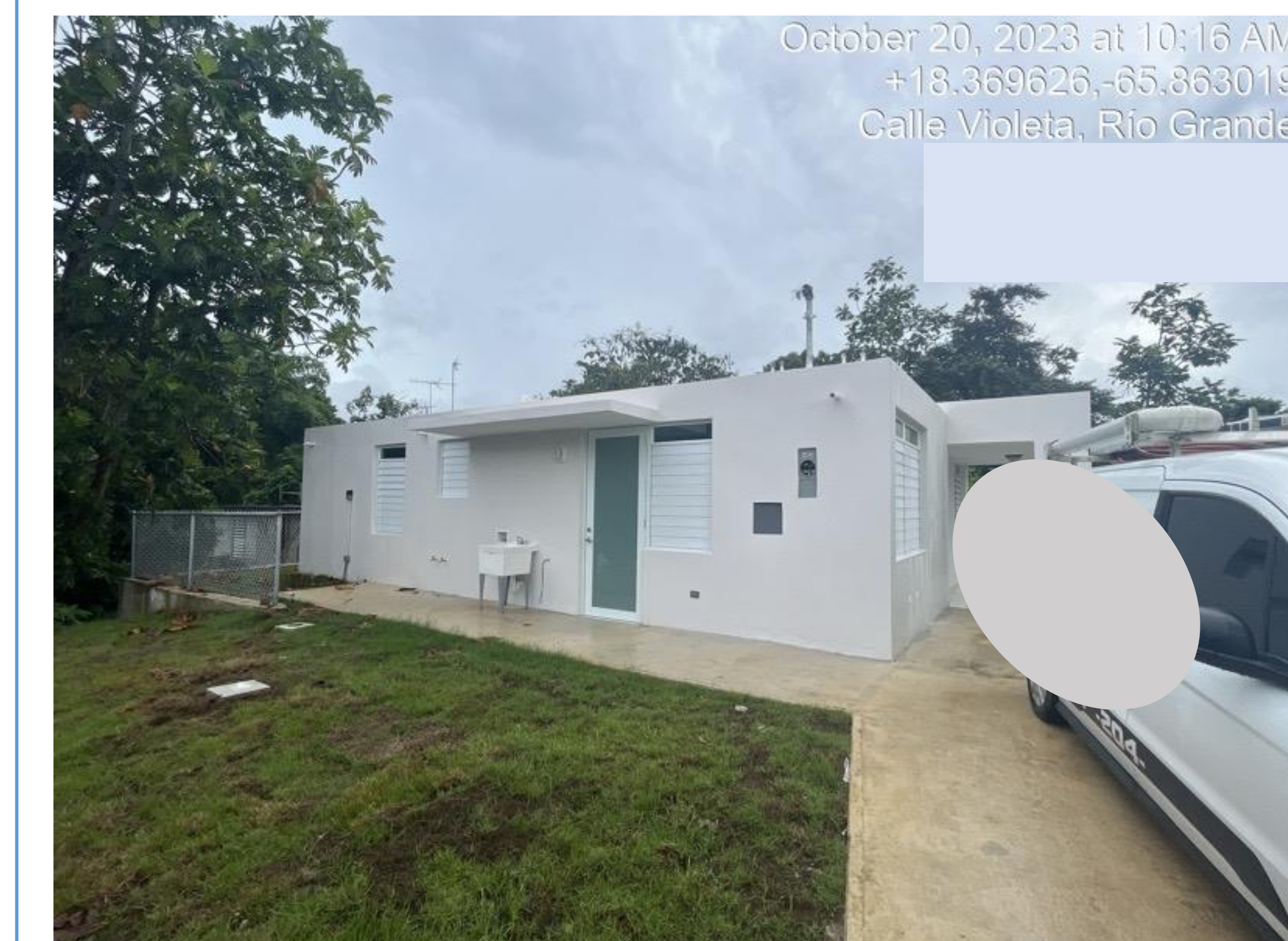
Figure 6. View of main entrance towards property site
