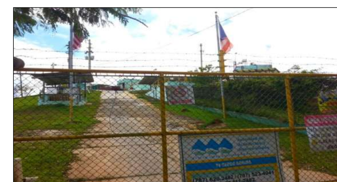
Fig. 2: Barrancas Filtration Plant
