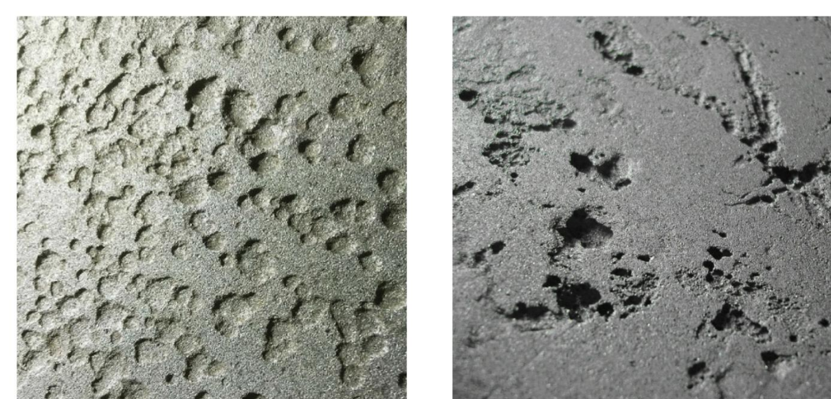
Source: Abfad, "Pitting Corrosion and Storage Tank Failure" https://www.abfad.co.uk/editorial/pitting-corrosion-and-storage-tank-failure/
